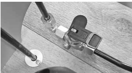
Shut-off valve for the heating system
